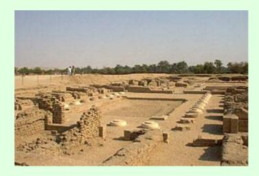
Since the new city of Akhetaten had to be built within a very short time, the traditional use of stone in the construction of royal buildings was replaced throughout by a type of brick known as *talatat*. This was smaller than the traditional stone block and therefore easier to transport and assemble.
